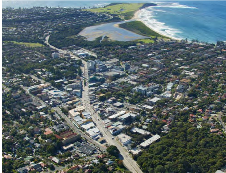
Figure 1 - Aerial photograph of the Dee Why Town Centre
